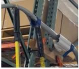
Manually or with the disengaged hotstick, support the opposite sleeve above the conductor while pulling the hotstick (still engaged in the attachment tool) along the conductor and away from the cap. Repeat on the other side.
