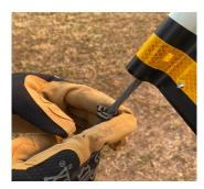
Place the retention clip around the wire underneath the marker and pre-engage by hand.
