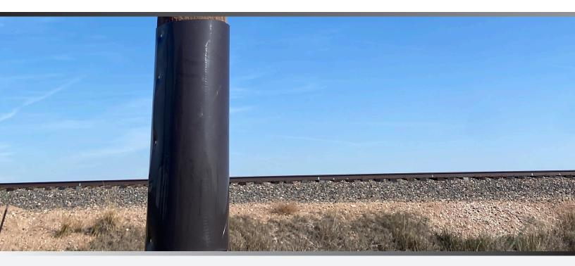
POLE WRAP IS A COST EFFECTIVE SOLUTION FOR REDUCING THE DAMAGE CAUSED BY CLIMBING ANIMALS AND WOODPECKERS.
