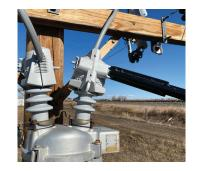
Position the bushing cover into place over the engergized equipment.
