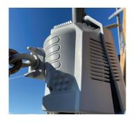
Adjust the fit by turning the eye screw clockwise until a tight fit has been achieved.
